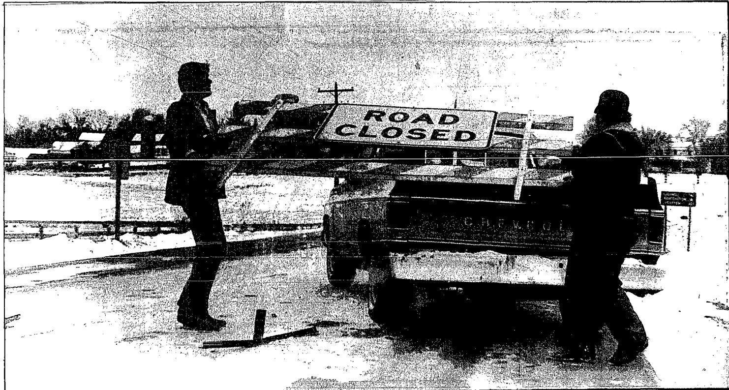
HOWARD STUBBENDIECK and Ken Palmer, both of Nider-Jergensen Construction Co., Omaha, toss state Highway 15's 'road closed' sign into the back of a pickup Friday morning.
